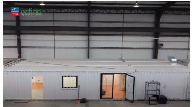
Figure 2: Construction of the factory in France, courtesy of CESI.
