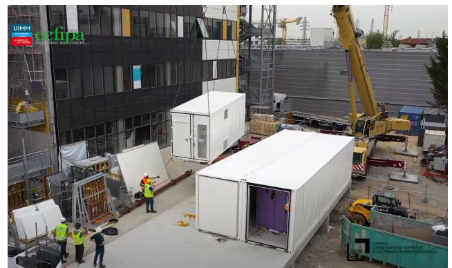
Figure 3: Installation of the factory at customer site, courtesy of CESI.
